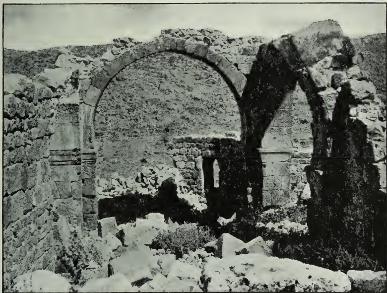
FIG. 284.—Viran Sheher 1, interior, looking towards apse.
